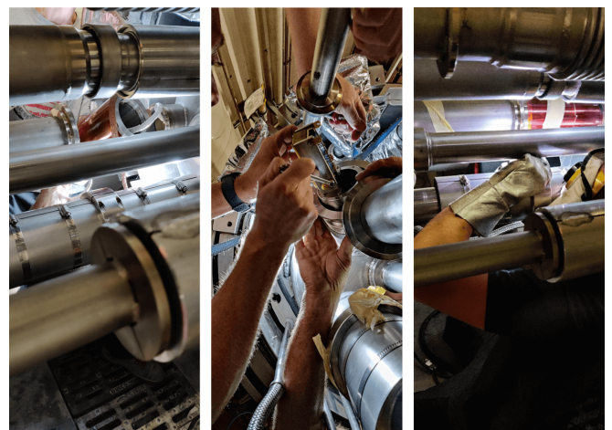
...MAKES THE DREAM WORK The new bellows were installed. On the far left: threading the instrumentation through the new bellows. In the middle: many hands make light work! On the right: skilled welders do their magic.
